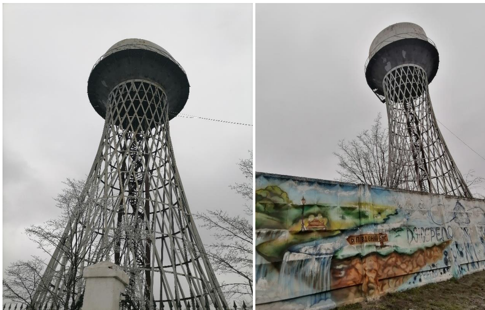
Fig. 1.11. Water tower and its strong frame (author's photo).
