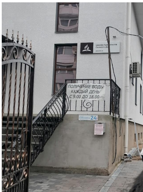
Fig. 1.29. A point for distributing purified water, equipped with a generator for uninterrupted operation in conditions of a power outage (photo by the author).
