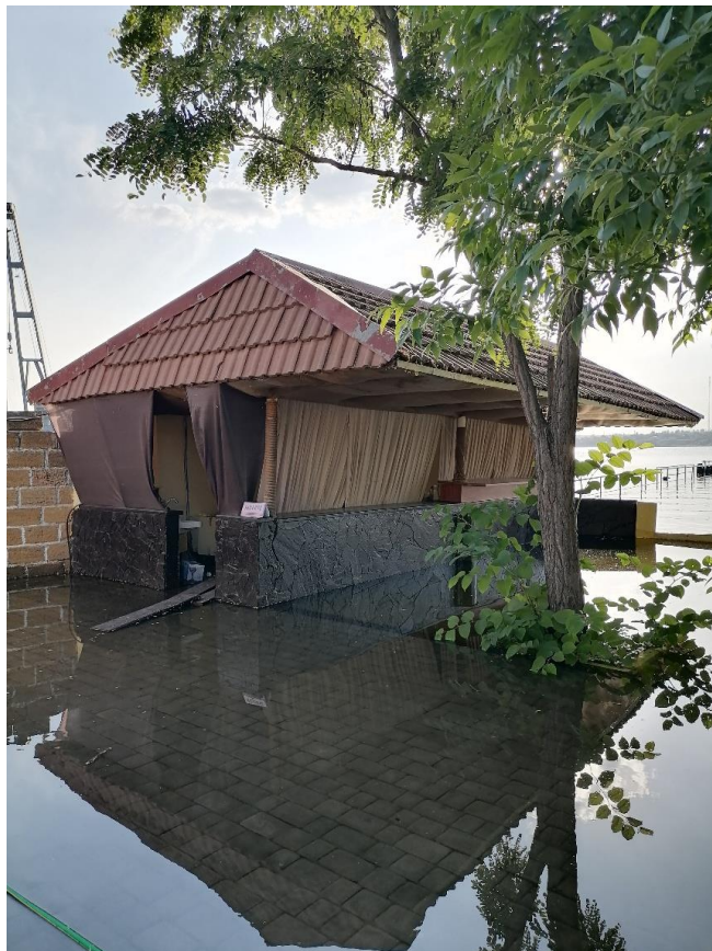
Fig. 1.28. "Venice" of the frontline city: flooded terraces of Mykolaiv (author's photo).
