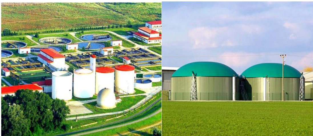
Fig. 4.31. Anaerobic digestion towers (upper figure municipal wastewater treatment plant for the city residence Petržalka of Bratislava capital where biogas production during sludge digestion process is combined with electricity co-generation unit).
