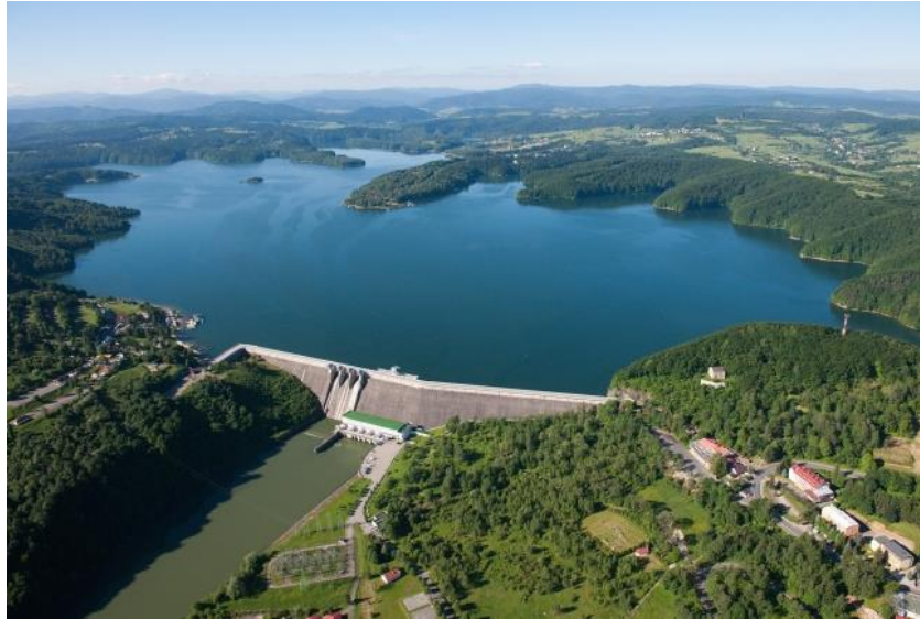
Fig. 3.2. Solina high retention reservoir. Below the dam, the power plant with the upper part of the Myczkowce equalizing reservoir (photo by L. Mnich)
