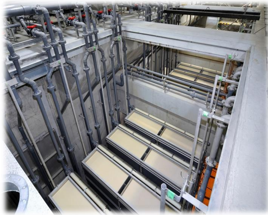
Fig. 4.20. Plate membrane reactor for N – microorganisms retention and high sludge age reaching (simultaneously cleaned using the air).
