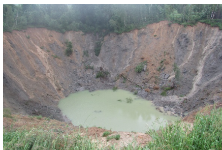
Fig. 8. Sinkhole No. 30 with a diameter of about 150 m immediately after the formation as of March 15, 2020
