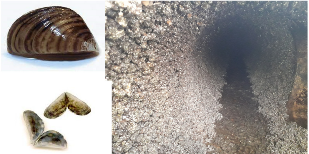
Fig.1. Zebra and Quagga Mussels colonising water intakes (Source: Bristol Water)
