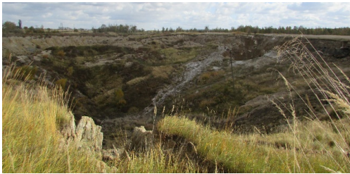
Fig. 5. Sinkhole on unit № 10 of South-East mine No. 2 of Stebnytsky Mining and Chemical Enterprise "Polymneral" in the area of chambers No. 108-113, which occurred on September 30, 2017
