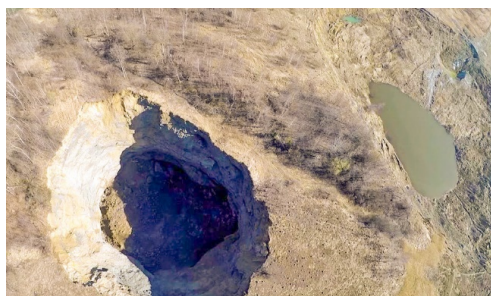
Fig. 7. Sinkhole No. 30 with a diameter of about 150 m immediately after the formation as of March 15, 2020
